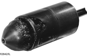
Figure 5-6. Typical Appearance of Flashing Damage
